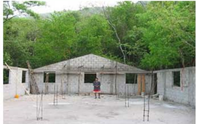
Classrooms under construction above church building in Oxtomal
