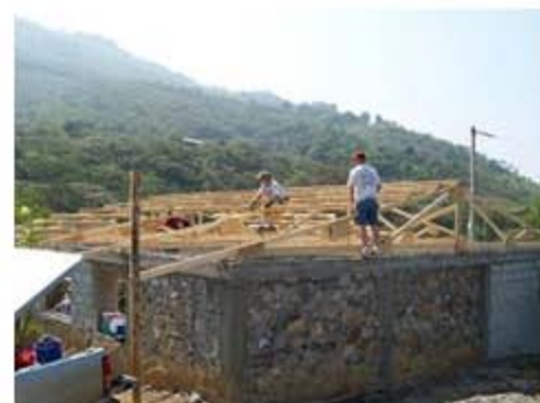
Brazospointe Fellowship laborers building new church roof in Tenango
