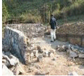
Hatchery construction in Totonicapá
